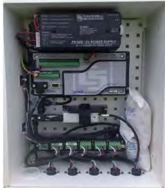
Datalogger for up to 5 SAA
